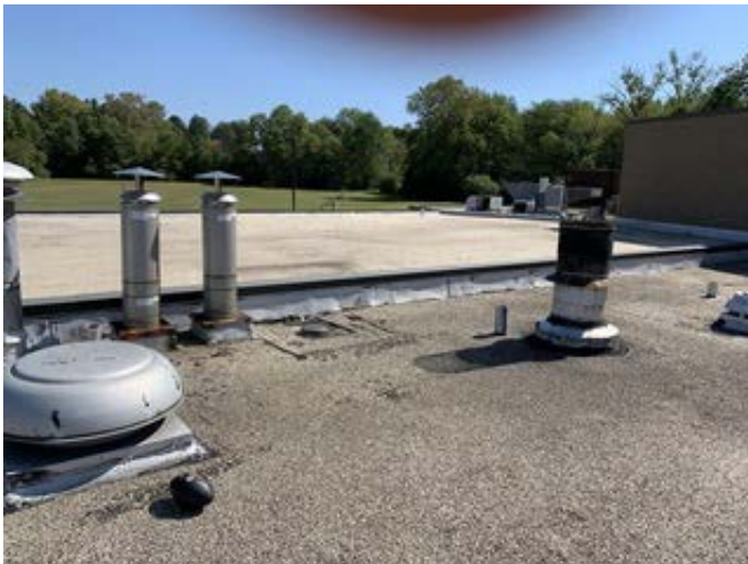
Ballasted Membrane Roofing
