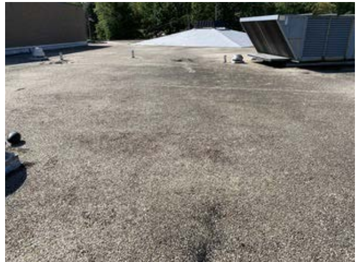
Ballasted Membrane Roofing
