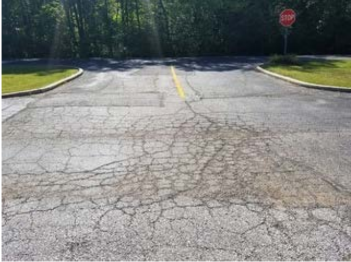
Cracked Asphalt
