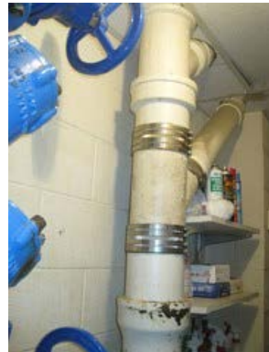
Cast iron sanitary piping
