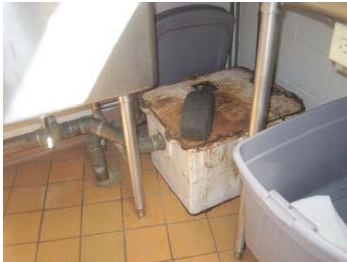
Grease waste interceptor
