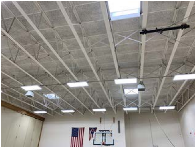
Steel Joists at Gym
