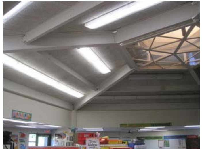
Surface-mounted LED lights in classroom
