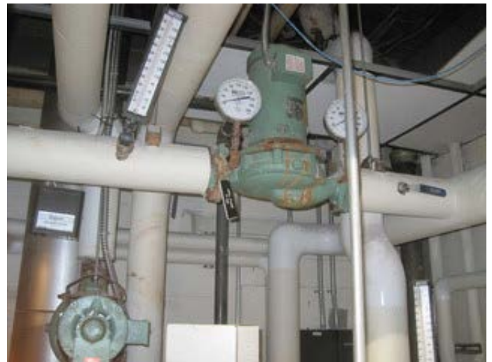
Heating system circulating pump
