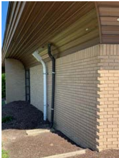
Metal Soffits & Brick Masonry
