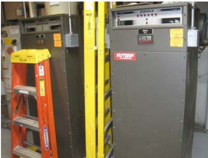
Heating water boilers
