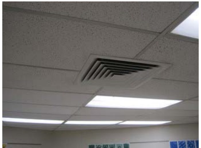
Air-distribution supply diffuser
