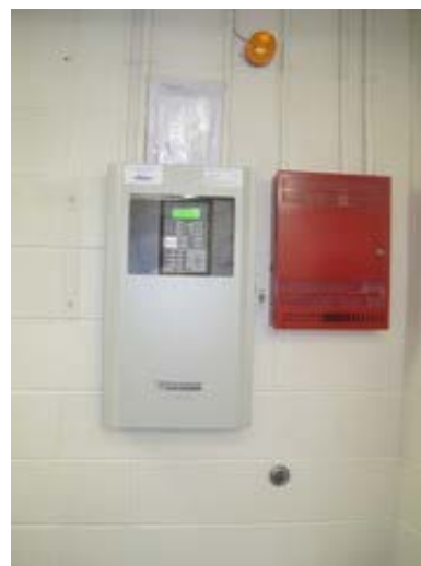
Main fire alarm panel
