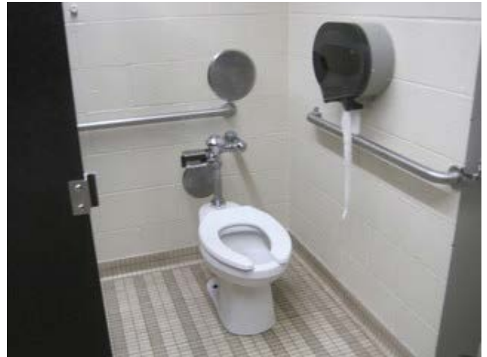
Floor-mounted water closet
