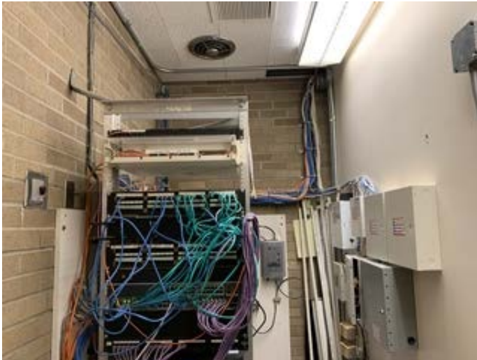
Main tech closet
