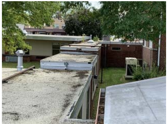
Ballasted Membrane Roofing
