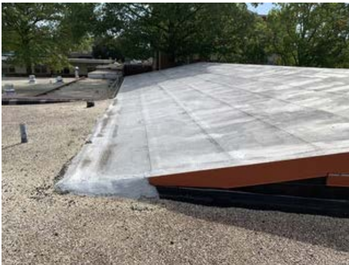
Ballasted Membrane Roofing
