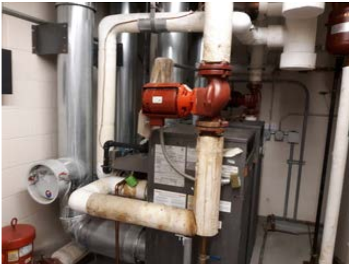
Boilers inside electric room
