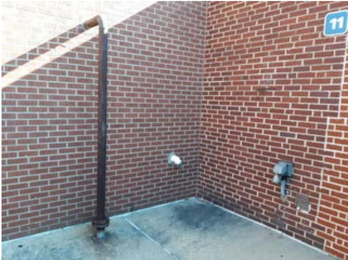
Portable generator plug
