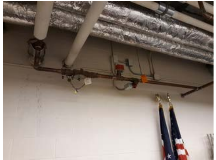
Limited area sprinkler piping
