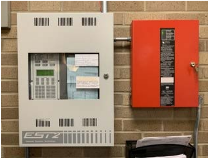
Fire alarm panel
