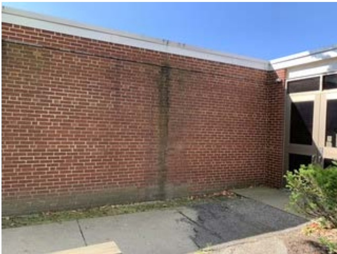
Brick Surfacing That Needs To Be Cleaned
