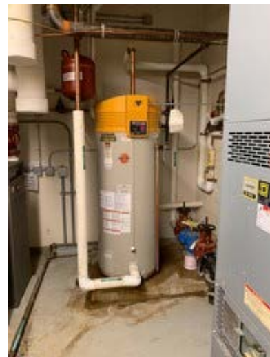
Water service entrance
