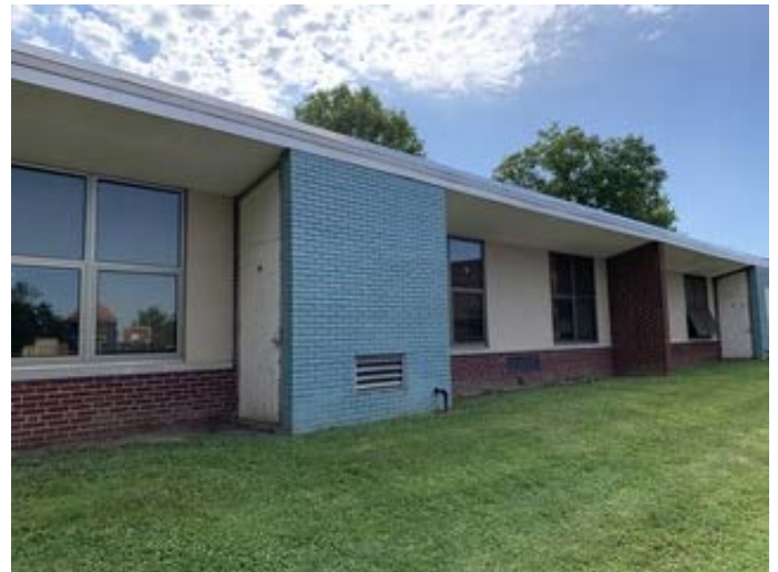
Exterior Doors - 1960 Building Addition
