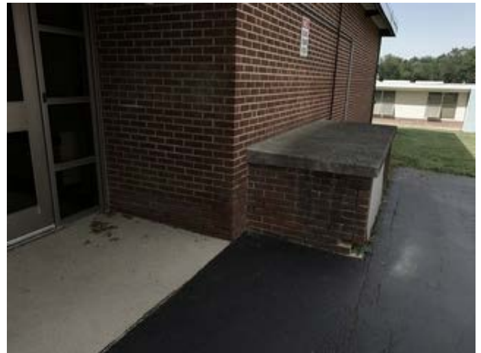
Brick Surface Needing Repair
