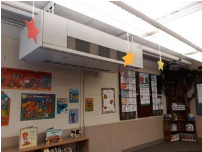
Unit ventilator in Library
