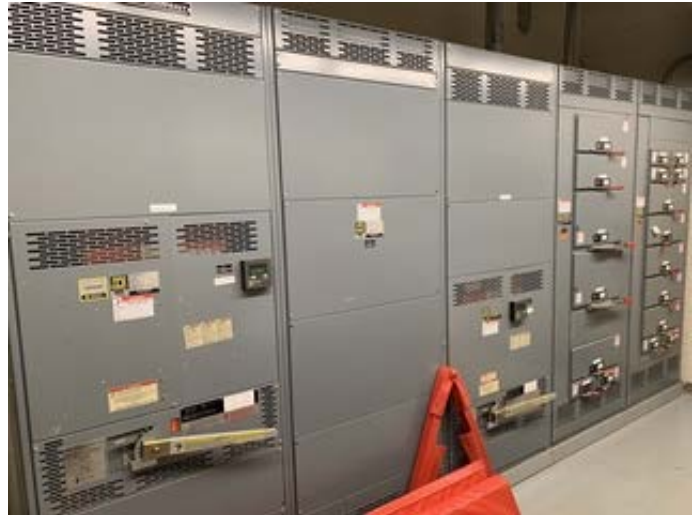
Main electrical service
