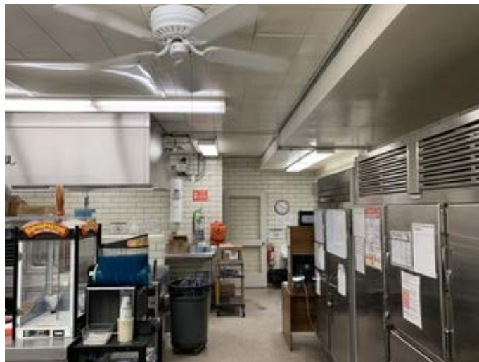
Kitchen hood extinguishing system
