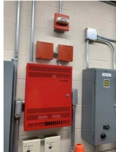
Wall strobe in electric room
