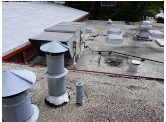
Kitchen make-up air unit
