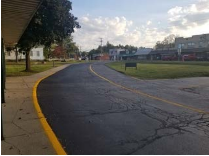
Cracked Asphalt
