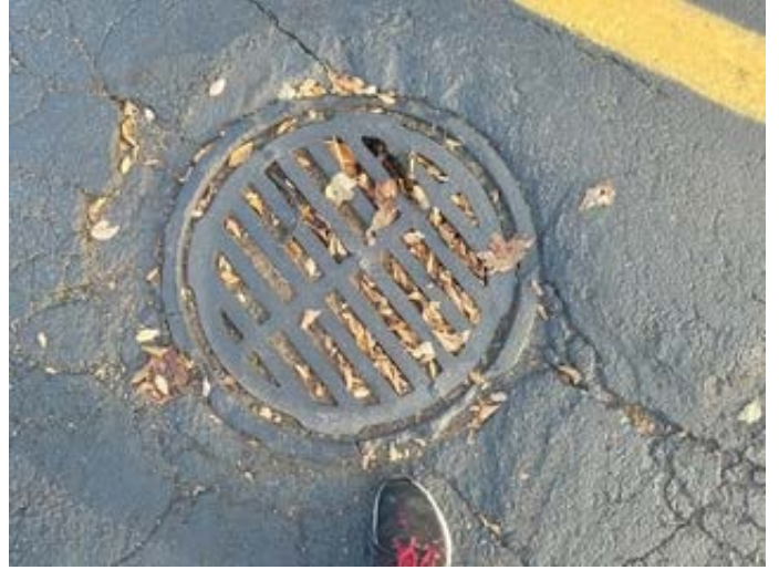
Debris Filled Catch Basin
