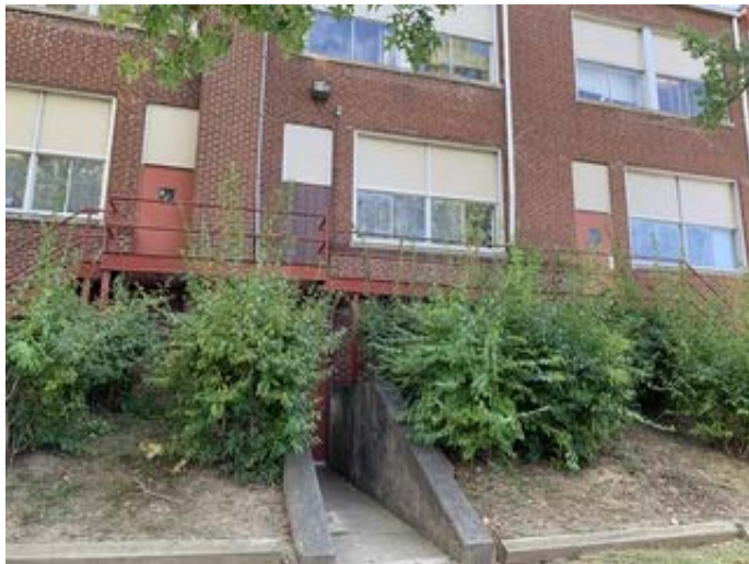
Exterior Doors - 1916 Building
