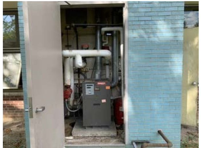
Boiler in outside room
