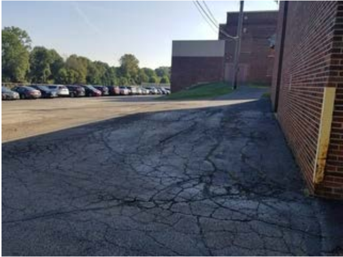
Cracked Asphalt
