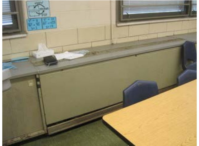
Classroom unit ventilator
