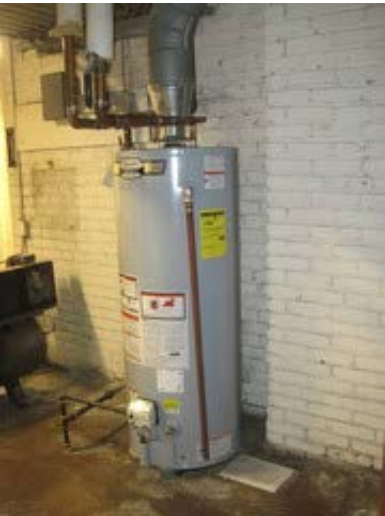
domestic water heater
