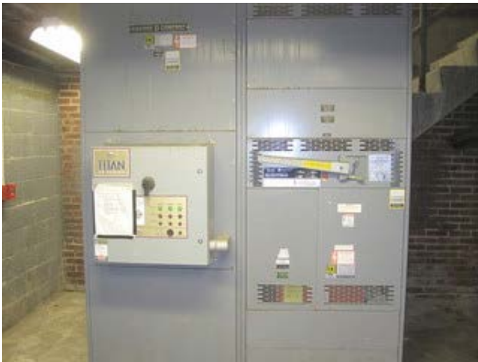
208/120-volt main switchgear
