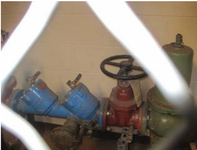
Domestic water BFP
