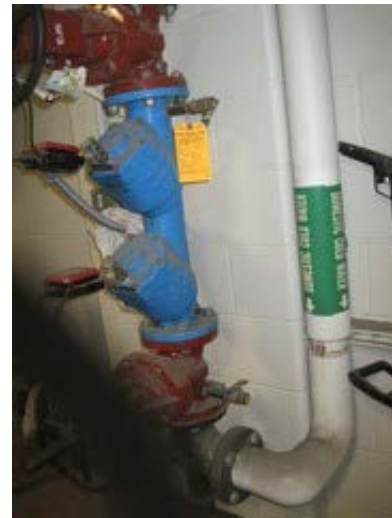
Main water service
