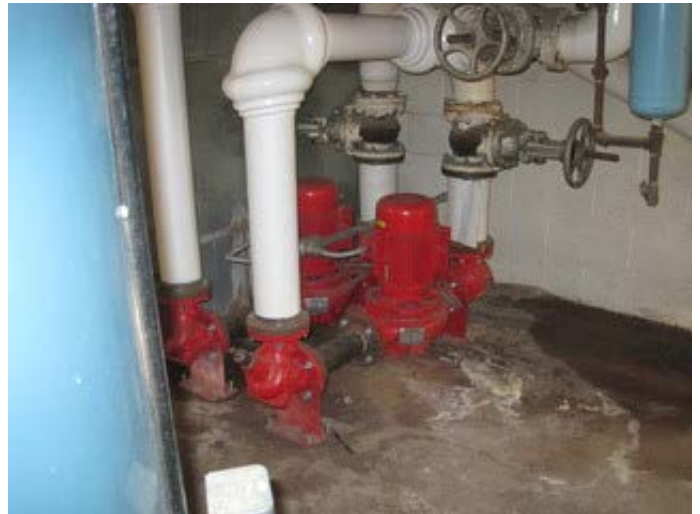
Heating water pumps
