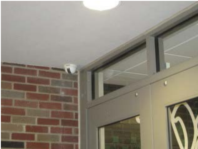
Main vestibule camera
