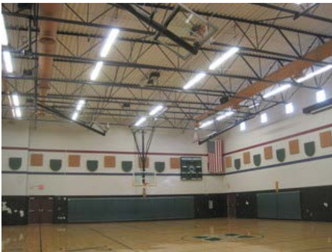
Gymnasium high-bay lighting
