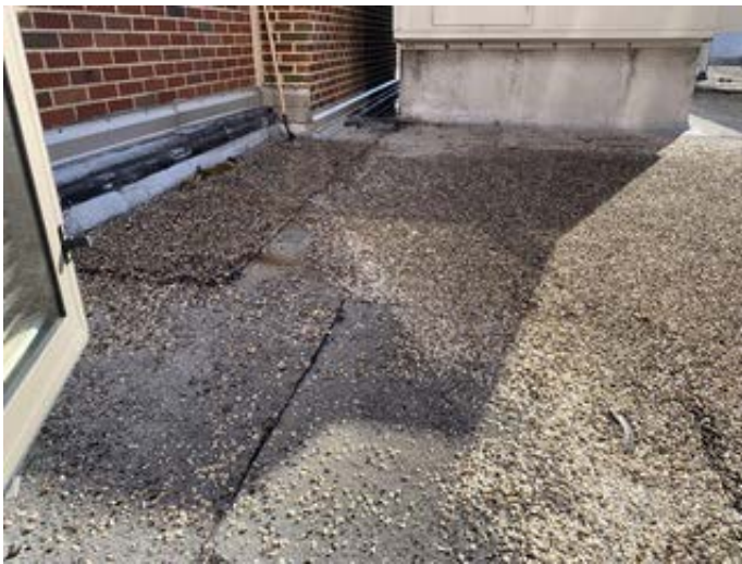
Ballasted Membrane Roofing
