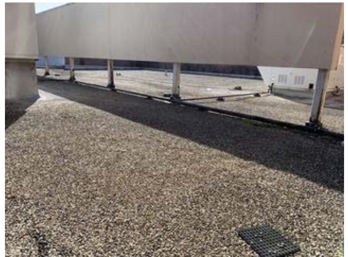
Ballasted Membrane Roofing
