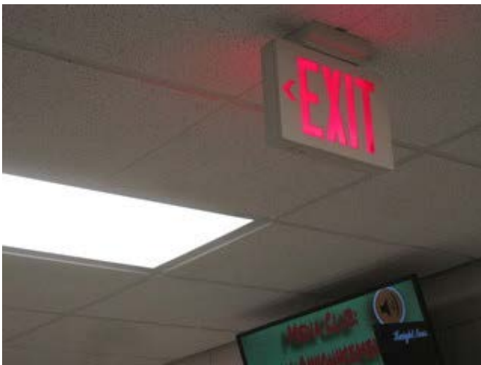
Typical exit sign
