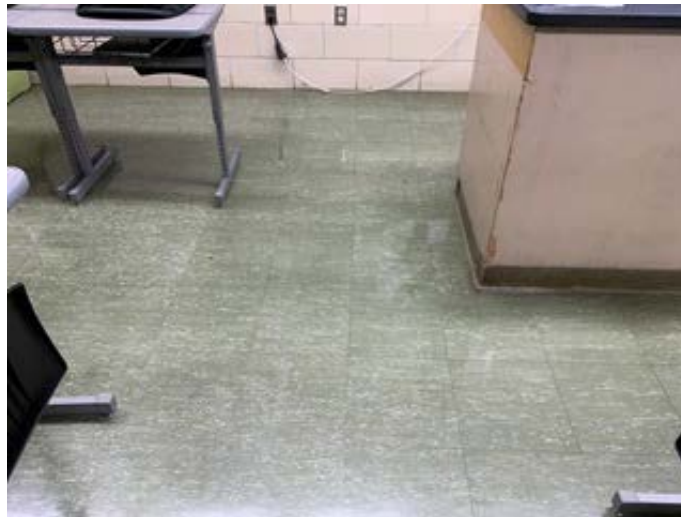
VAT in a Classroom
