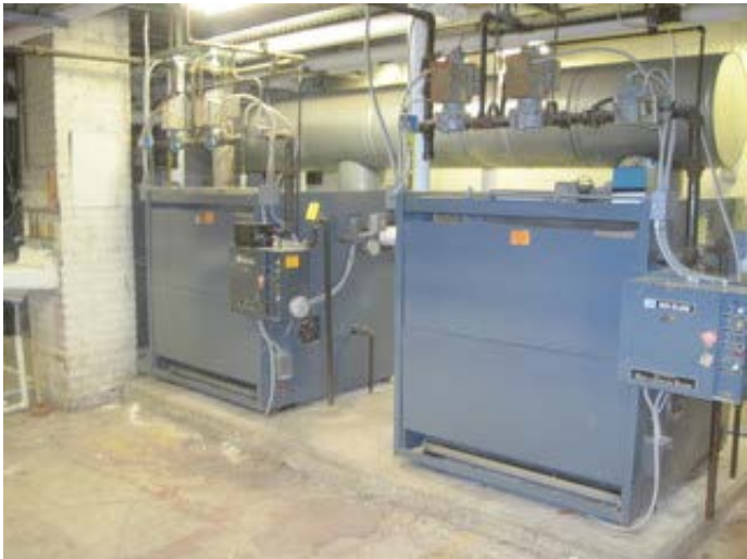
Heating water boilers
