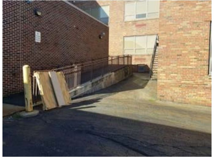
Non-compliant ADA Ramp
