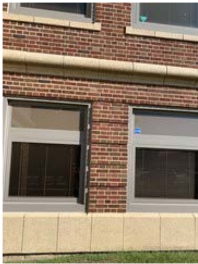
Close Up of a Typical Window
