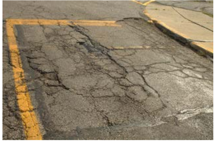
Failing Asphalt and Curb
