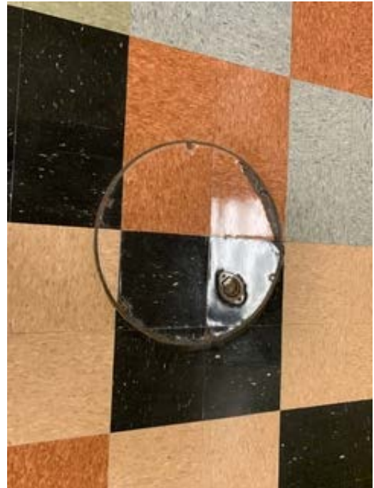
Acid neutralization basin
