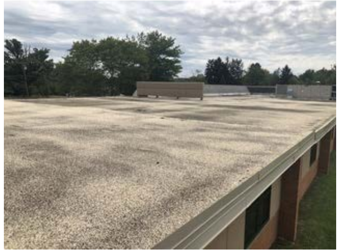
Ballasted Membrane Roofing
