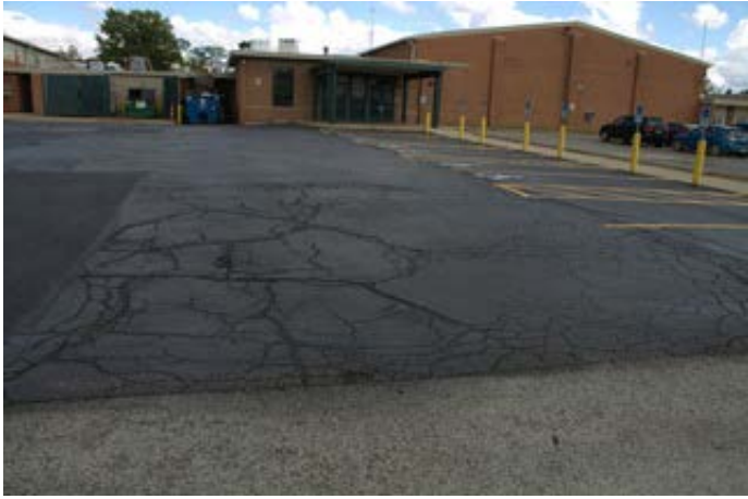
Cracked Asphalt
