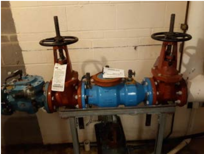
Meter backflow preventer
