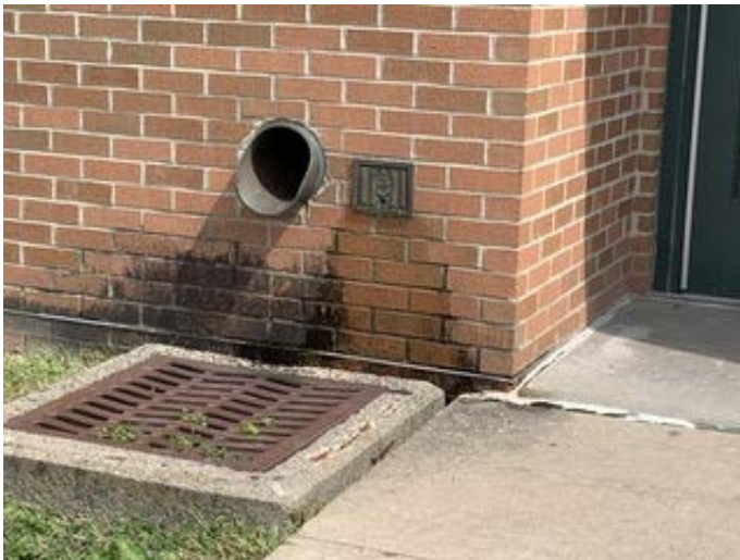
Masonry That Needs To Be Cleaned
