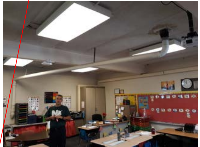
Added roof drain
