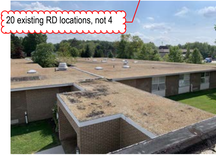
Ballasted Membrane Roofing
