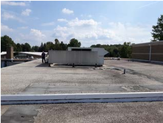
Rooftop VAV unit
