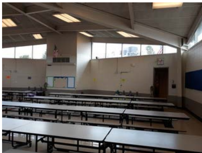
Cafeteria exit lights
