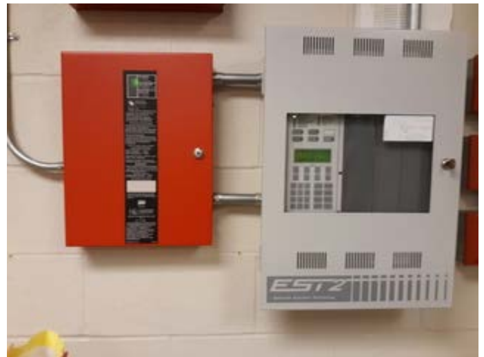
Fire alarm panel
