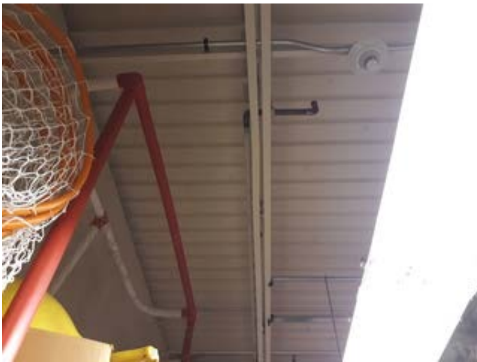
Limited area sprinkler head
