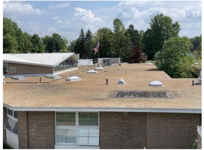
Ballasted Membrane Roofing
