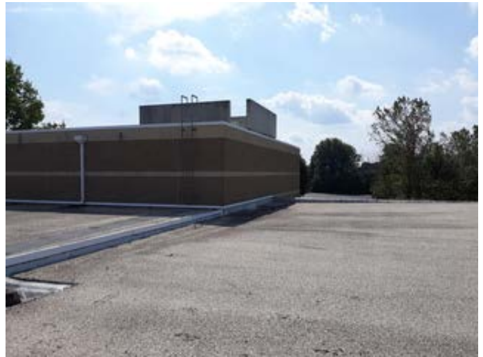
Gym HVAC unit
