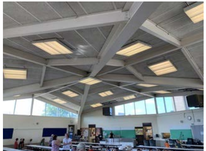
Steel Beams at a Classroom
