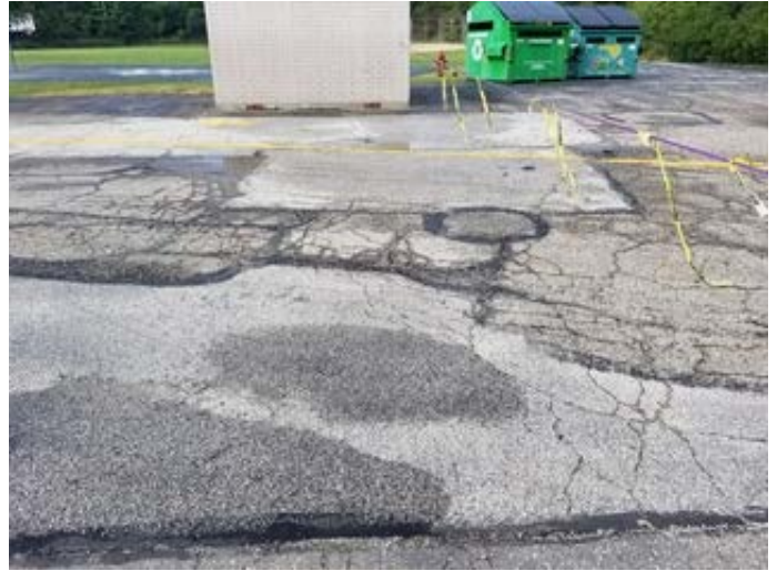
Cracking Asphalt
