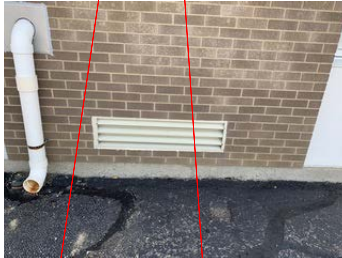
Masonry Infill at Unit Ventilators
